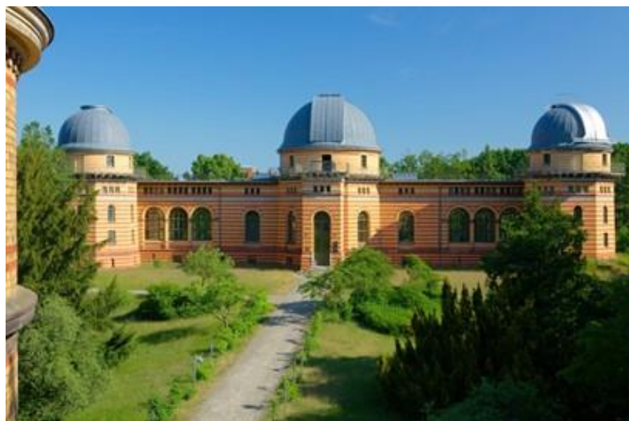
Fig. 1. Main building of the Astrophysical Observatory Potsdam.
