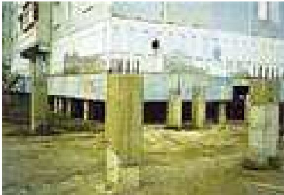
Buildings on piles in permafrost
