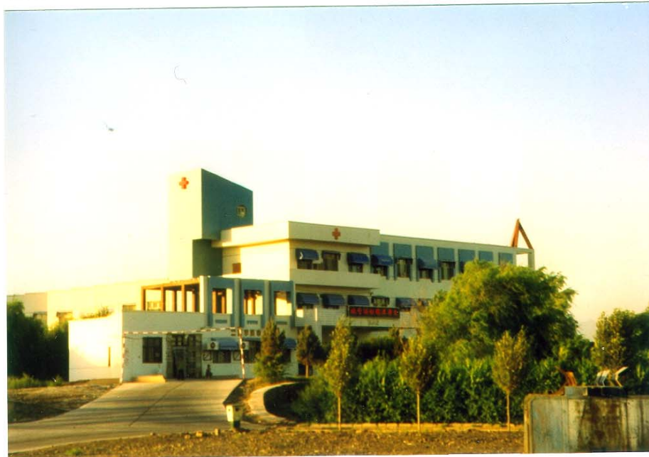
Bild 19: Sanashan Railway Station, Krankenhaus
